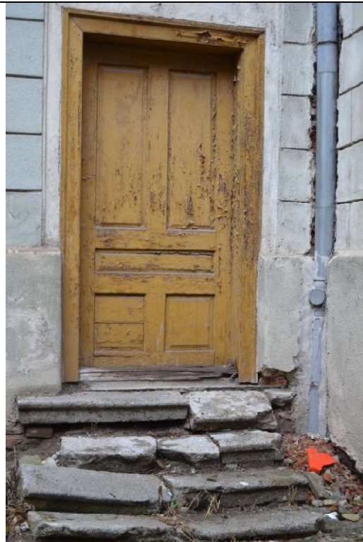
TRONSON C –PARTER ACCES INZIDIT SPRE CORIDOR
