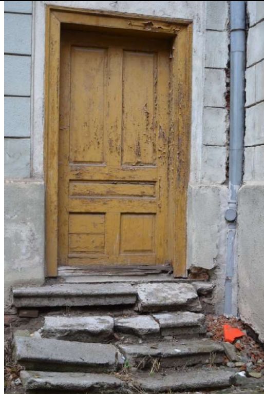
TRONSON C –PARTER ACCES INZIDIT SPRE CORIDOR
