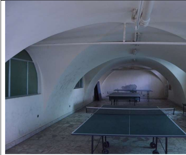
TRONSON A - SUBSOL, BOLTA CILINDRICA, ARC CURBURA VARIABILA
